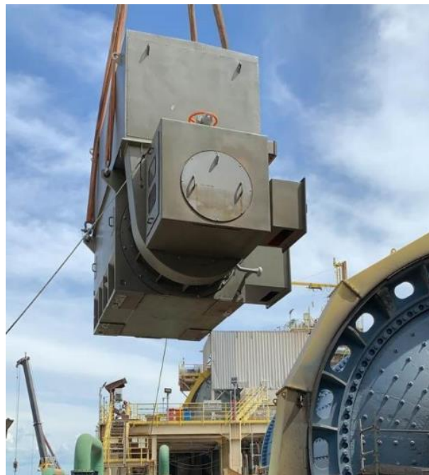
Installation of repaired motor on ball mill
