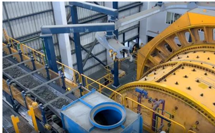
ZEP radial stacker and SAG mill hot commissioning – November 2020
