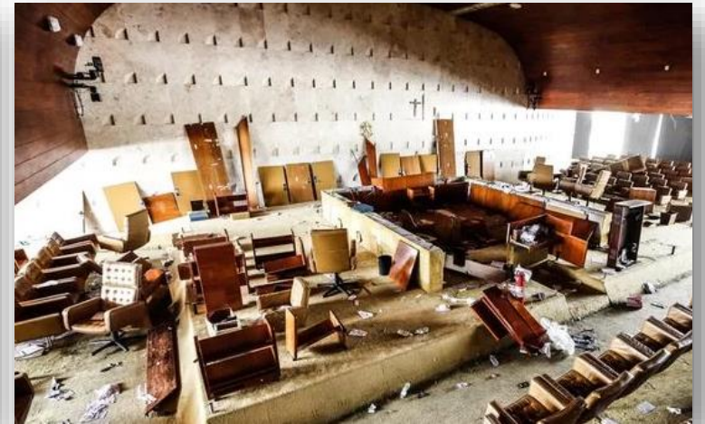
Supreme Court Plenary Room
